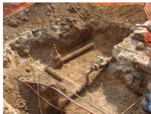
Above: Unmetered and metered supplies exposed. (© WRP (pty) Ltd)
