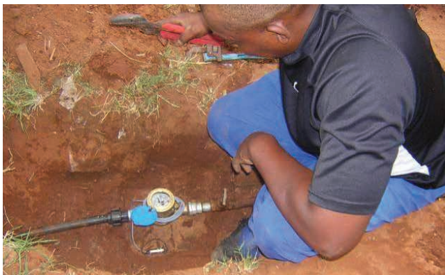
Above: Installation of a loggable consumer meter (© WRP (pty) Ltd.)
