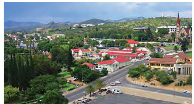
Above: Covered reservoirs and greenery maintained with purified effluent in Windhoek (© WRP (pty) Ltd)
