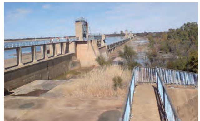
Above: Start of a 113km canal in the Lower Vaal River Catchment (© Vaalharts Water User Association)
