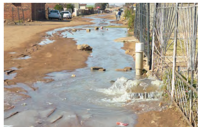
Above: Burst pipe in Evaton (© Morena Mokubung)
