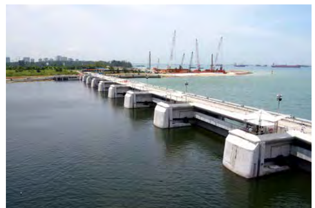
Above: The Singapore Marina Barrage creates a freshwater reservoir keeping out seawater (© ngotoh - Flickr)
