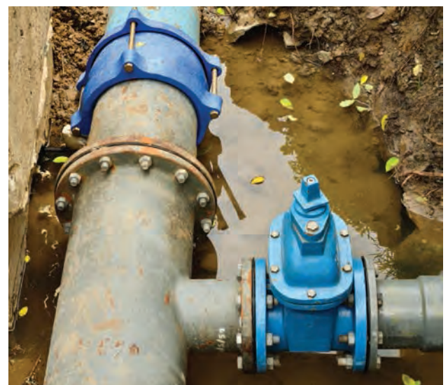
Above: Upgrades to domestic water supply pipe work (© Pupunkkop | Dreamstime.com)
