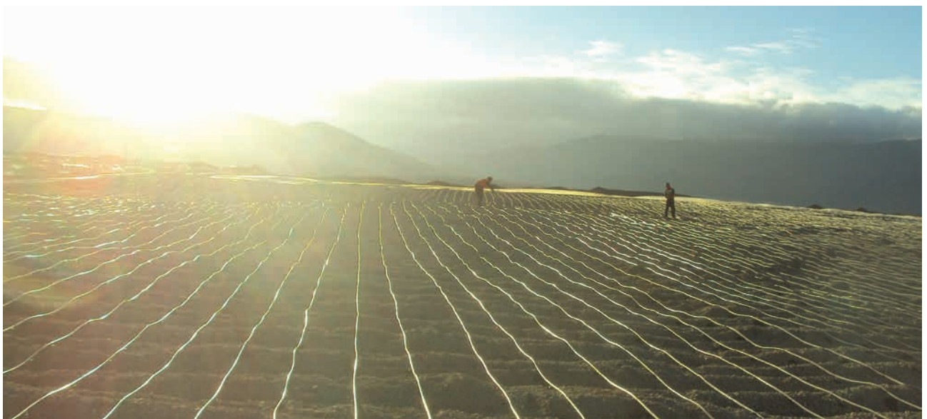
Above: Leach Pad irrigation system (© Xstrata Copper)
