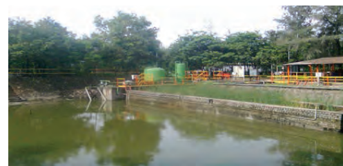
Above: Reuse of blowdown water for horticulture; Water collected in swale for reuse (© Bharatendu, D)
